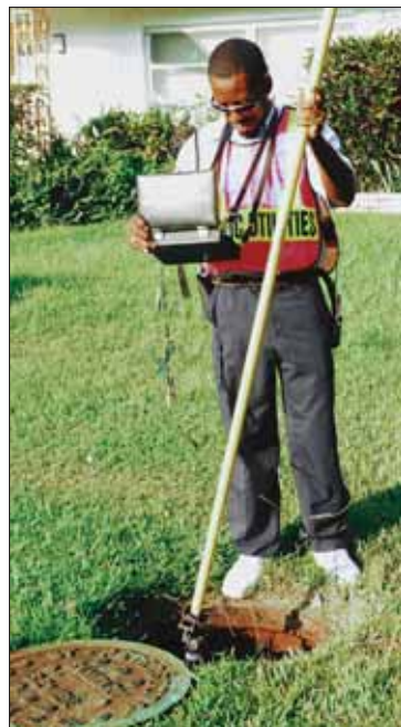
Above, the Quick Television crew from the city's Preventive Maintenance Section uses a pole camera to inspect sewers. Operating the camera is wastewater technician DiMario McKenzie. Right, wastewater technician John Martin cleans a line as wastewater collections system maintenance division manager Lane Longley observes.
