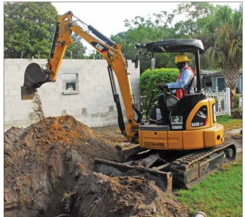
The Corrective Maintenance Repair crew uses a mini-track hoe to excavate a problem line and install a new section of PVC pipe.
